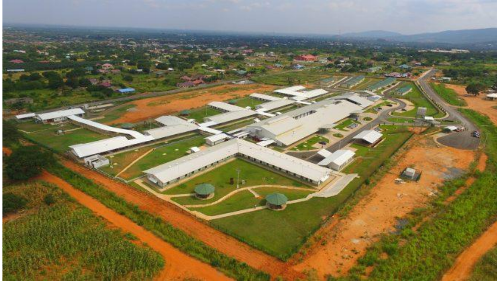
Ghana's Shai Osudoku District Hospital, Dodowa, Ghana by NMS Infrastructure
